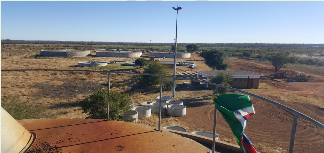
Warmbarths Waste Water Treatment Plant
