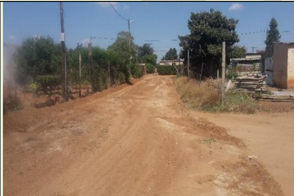
Routine road maintenance
