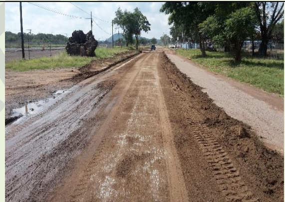
Grading of unpaved roads
