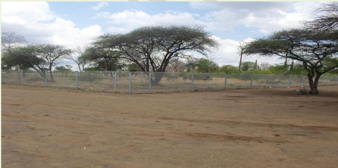
PICTURE:1 COMPLETED CLEAR VIEW FENCING AT THE CEMETERY ON THE R516 ROAD
