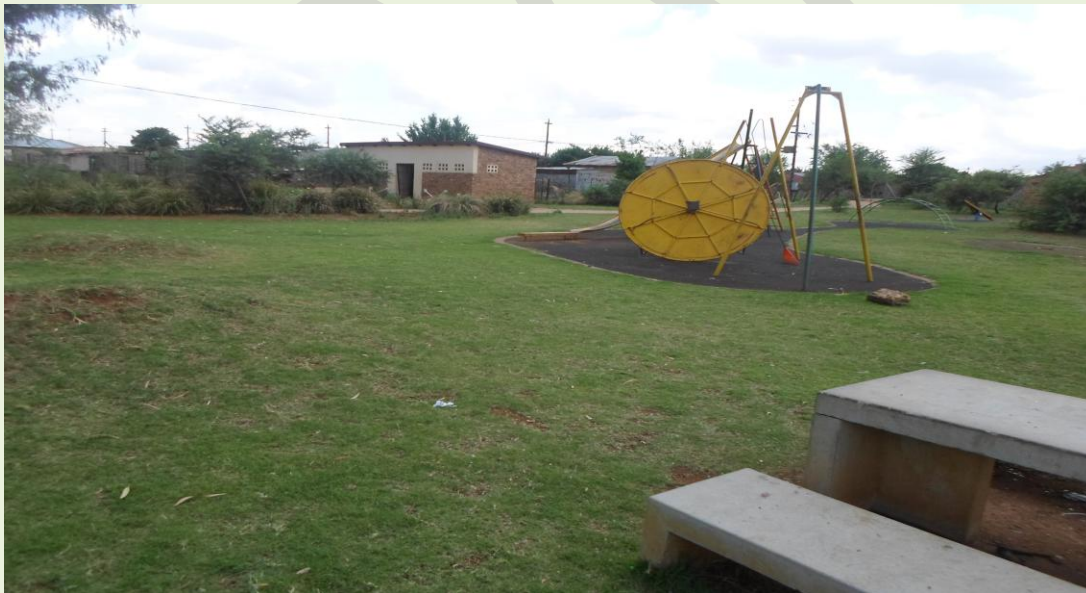
PICTURE: 10 ABLUTION FACILITIES AT PIENAARSRIVIER PARK
